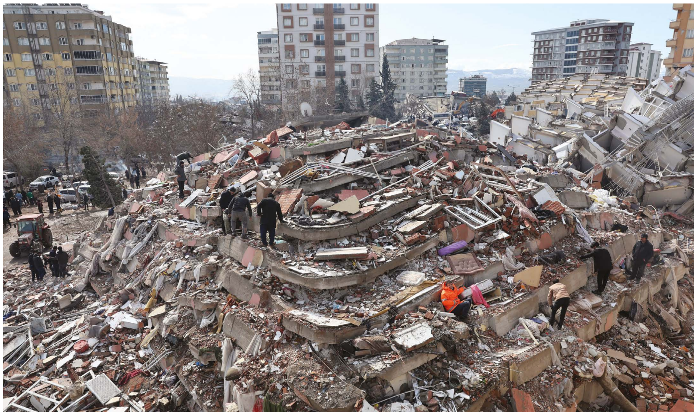
The magnitude-7.8 earthquake in Turkey last month destroyed many buildings, such as this one in the city of Kahramanmaraş.
