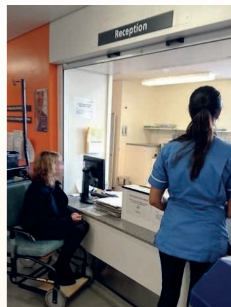
Fig. 5 Reception area with lowered portion
